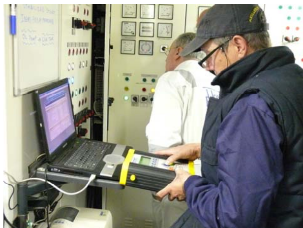
Hand Held Terminal in use during a real test
